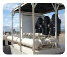
Instead of a single, large horsepower pump, Lindsay recommended Ochoa install three 100 horsepower (101.38 metric hp) pumps for variable demand needs and more efficient start-up. This recommendation was based on the ability to dynamically sequence the motors on the three pumps, which provides consistent water delivery and saves energy.
